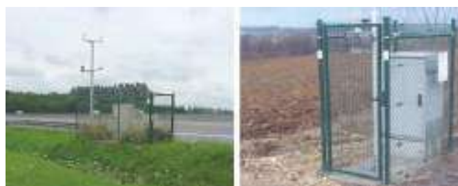
Primary RWS (left) along a Flemish road and secondary RWS (right) along a Walloon road
