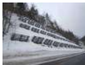
Avalanche control fence
