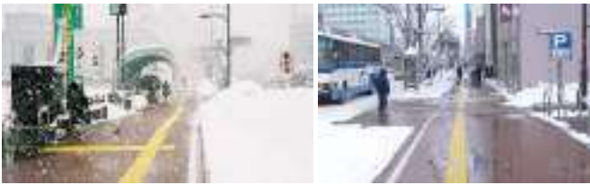
Snow melting with the system
